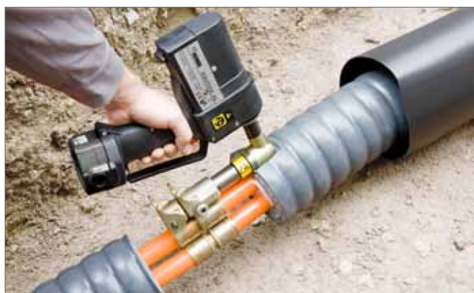
Afb. 2. RAUVITHERM schuifhulsverbinding
